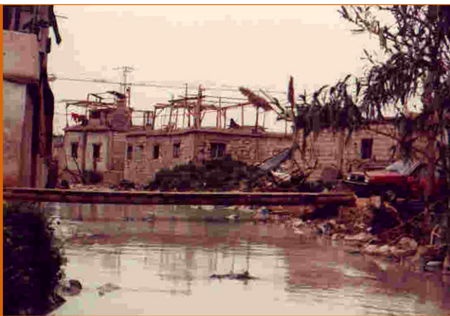
Environmental and physical degradation in Havy el Sellom
