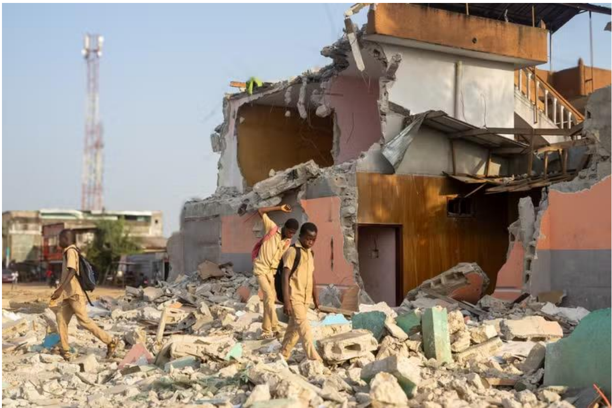
Figure 4: Schoolboys walk among the rubble left the Gesco quarter of Abidjan after the demolitions of the previous week, 26 February 2024. Source: Marine Jeannin/ Le Monde .
