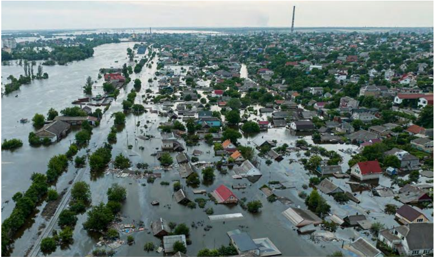
Figure 15: Flooding of the Dnipro River after the Kakhovka Dam breach. Keystone/AP.
